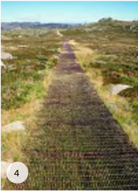
Selection: Heelsafe expanded walkway mesh Supplier: Total Steel
