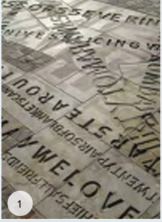
Selection: Sunset Gold Granite Details: 80mm thk Supplier: Sam the Paving Man
