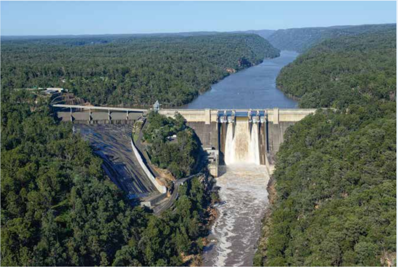
Warragamba Dam spilling, March 2021 Source: INSW Image: Adam Hollingworth
