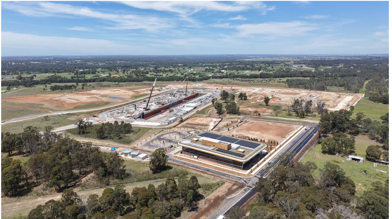
Bradfield City Centre under construction, Bradfield Development Authority
