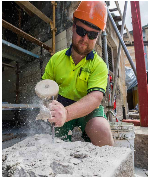
∨ Sandstone repairs, Parramatta North
