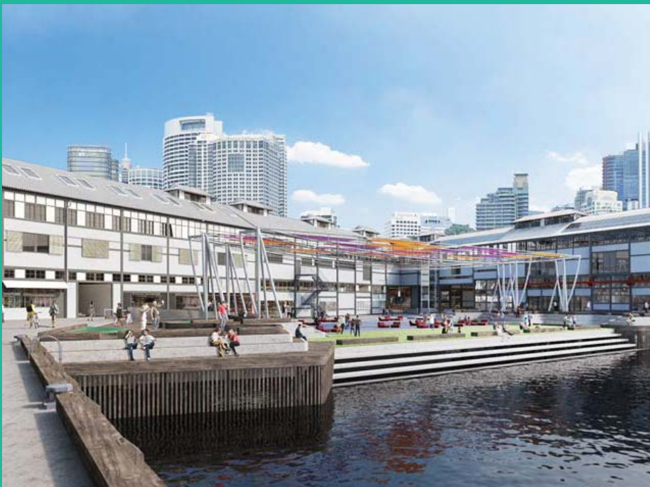
View from Pier 2/3 ground floor view
