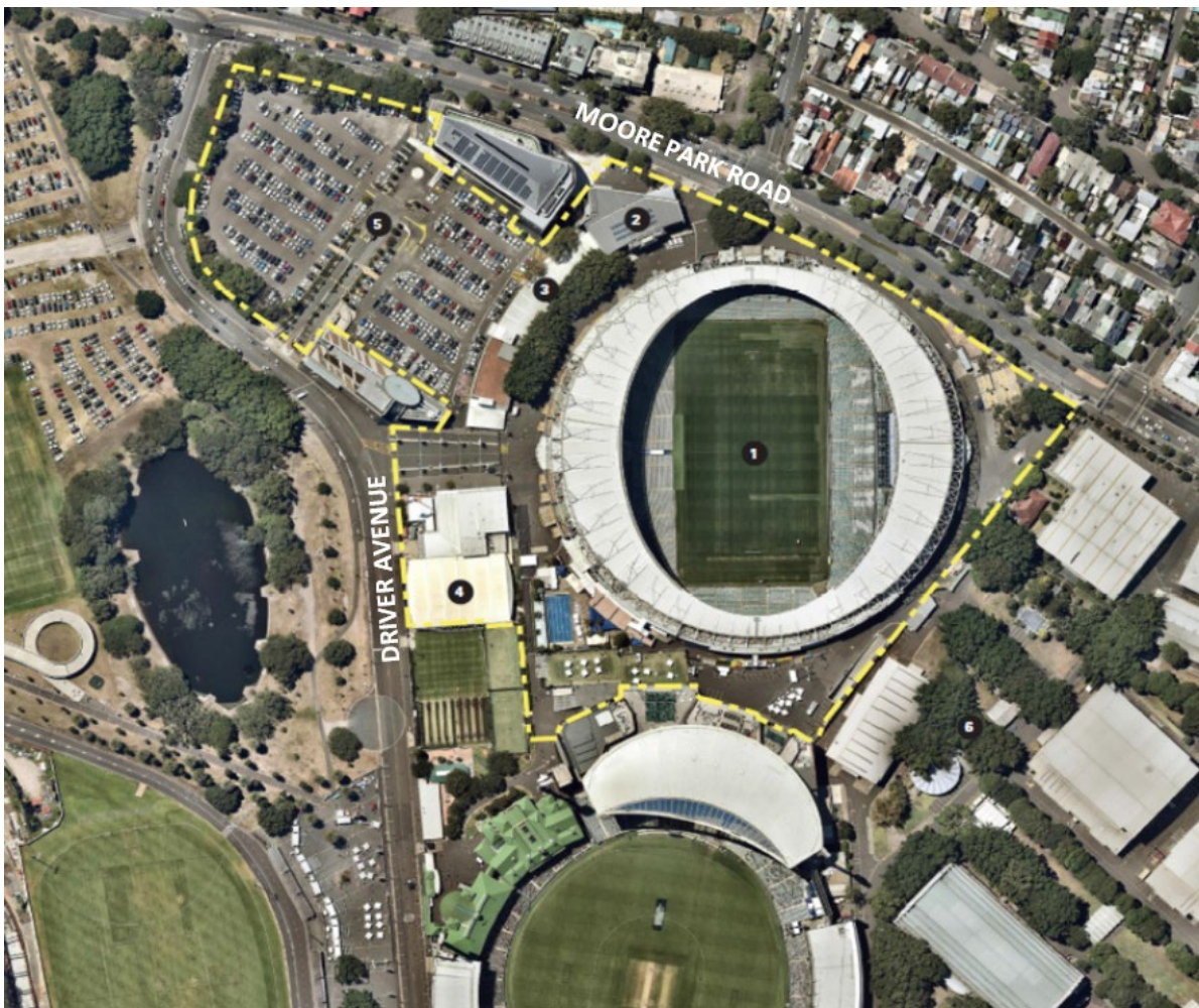
Figure 1: Site boundaries: 1: Allianz Stadium, 2: Sheridan Centre, 3: Sydney Roosters, 4: Cricket NSW, 5: MP1 Carpark
